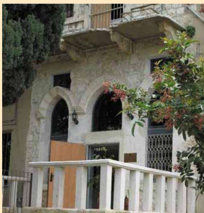
Top and middle: The El-Carmel Center under construction. Above: The finished building facade.
